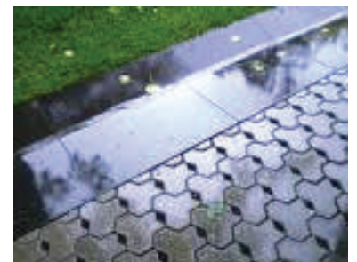
Permeable paving is one component of WSUD
